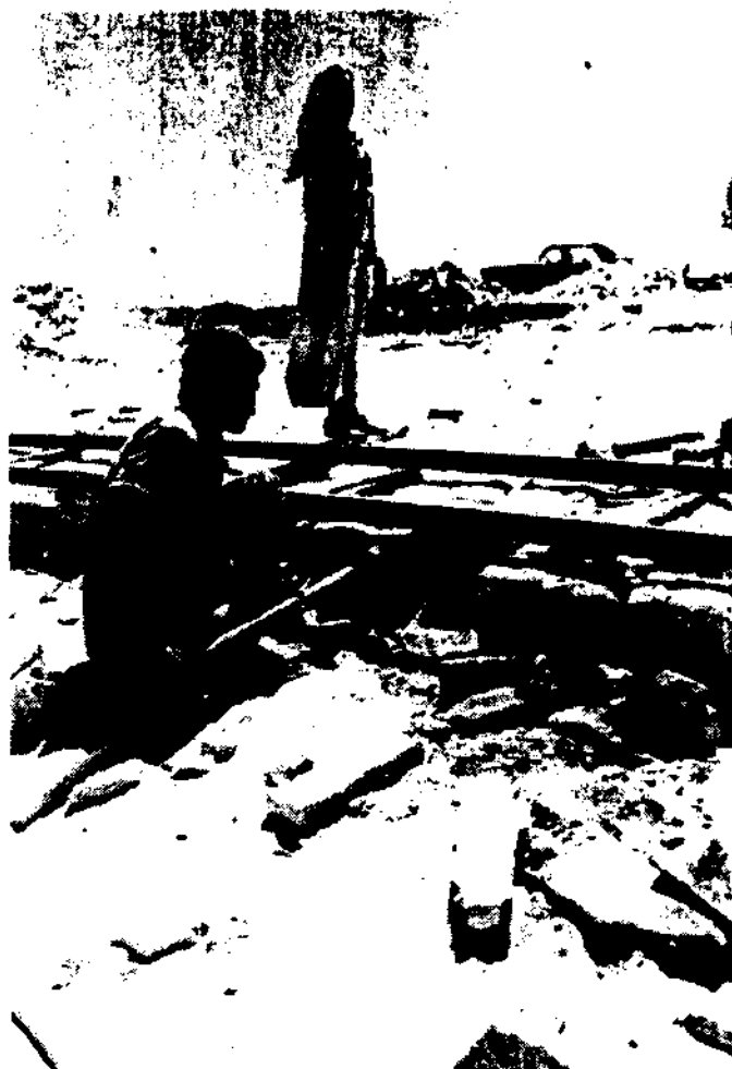
Fig. 822 Block is cut horizontally using the traditional method
