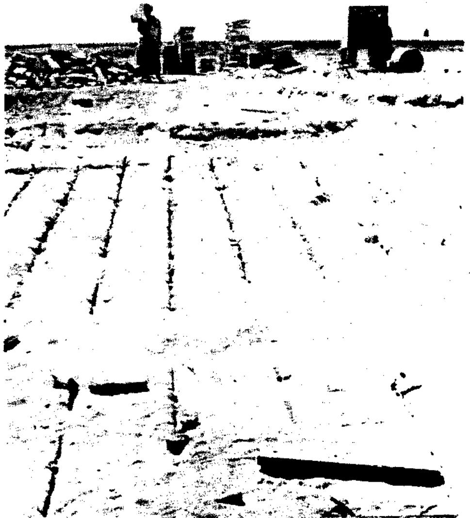
Fig. 821 The machine cuts parallel lines, then lines perpendicular to these
